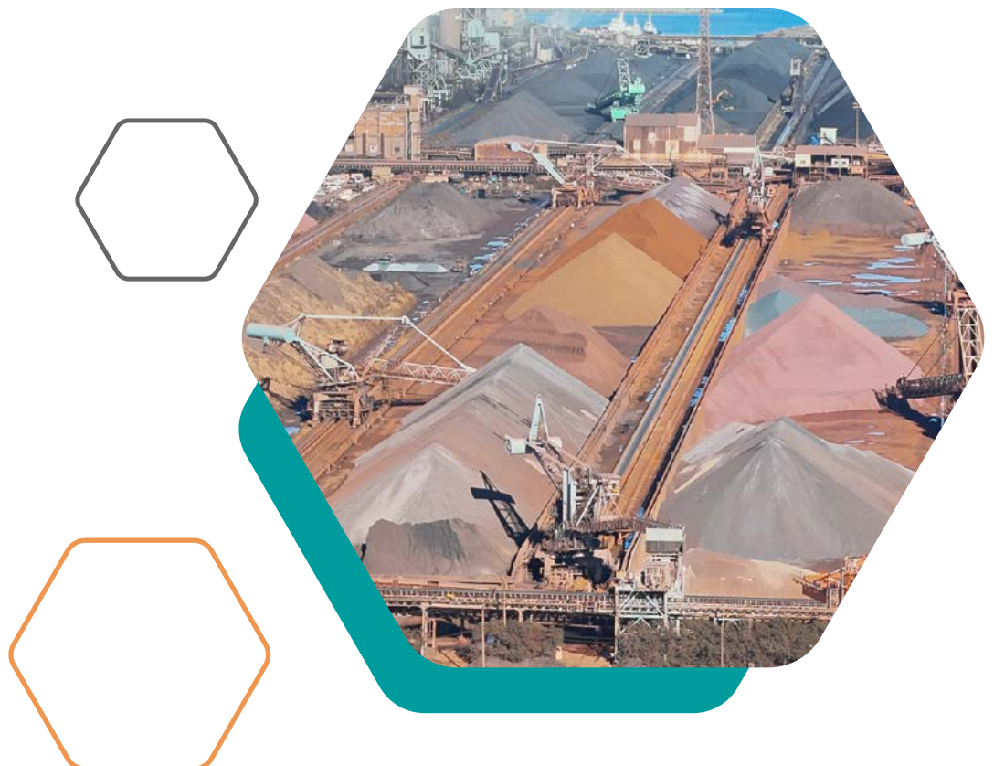
Nippon Steel's East Japan Works, Kashima steelworks. SteelWatch / FINE Co.,Ltd.
